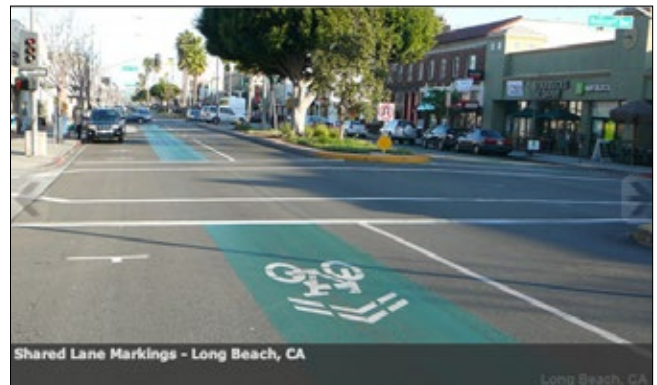
Shared lane markings ("sharrows"): Long Beach, CA
